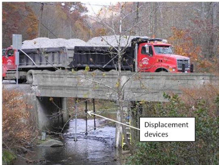
Figure 1.2: Static Bridge Testing
